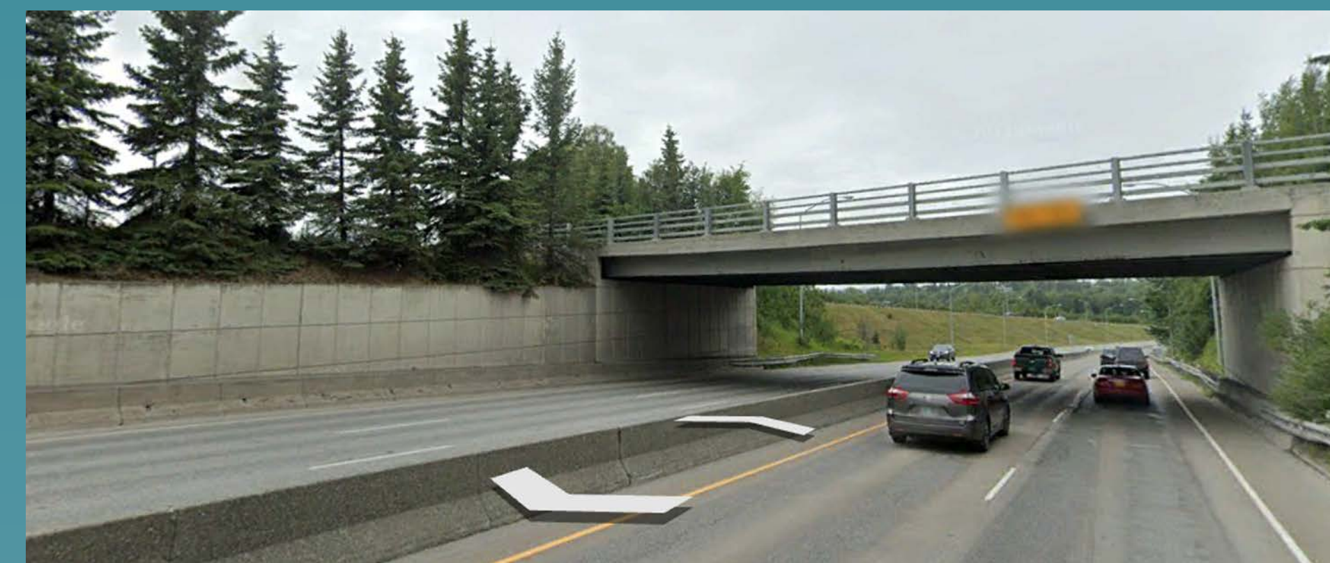
Minnesota Boulevard, Anchorage
