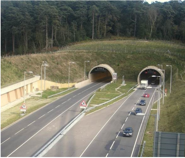
Figure 4. Side-by-Side Tunnel Example
