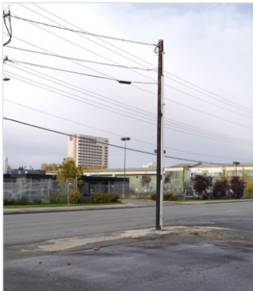
Utility Pole in Sidewalk.
